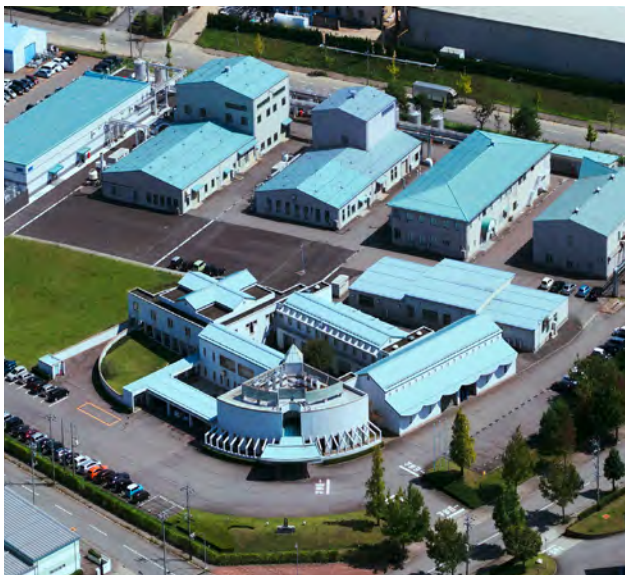
YMC Co., Ltd. manufacturing facility in Komatsu, Japan
